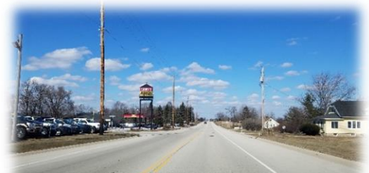
Wide Shoulder Heading into West Bend
